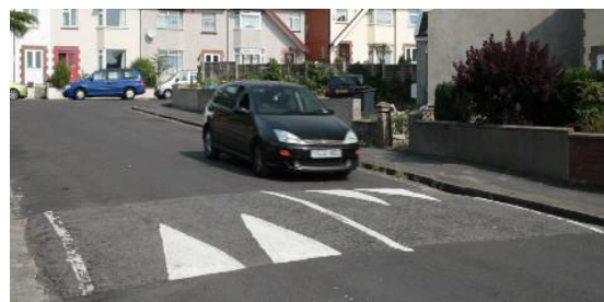
Fig3:humps on roads
